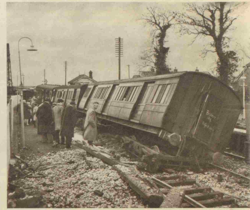
THE DAMAGED CARRIAGES OF THE EXPRESS TRAIN WHICH CRASHED AFTER JUMPING THE TRACK AT RUSH AND LUSK STATION ON JANUARY 5, AND BLOCKED THE BELFAST-DUBLIN LINE. OF THE TWO HUNDRED PASSENGERS ON THE TRAIN ONLY TWO WOMEN NEEDED TO BE HOSPITALISED: ONE FOR SHOCK AND THE OTHER FOR MINOR CUTS.
