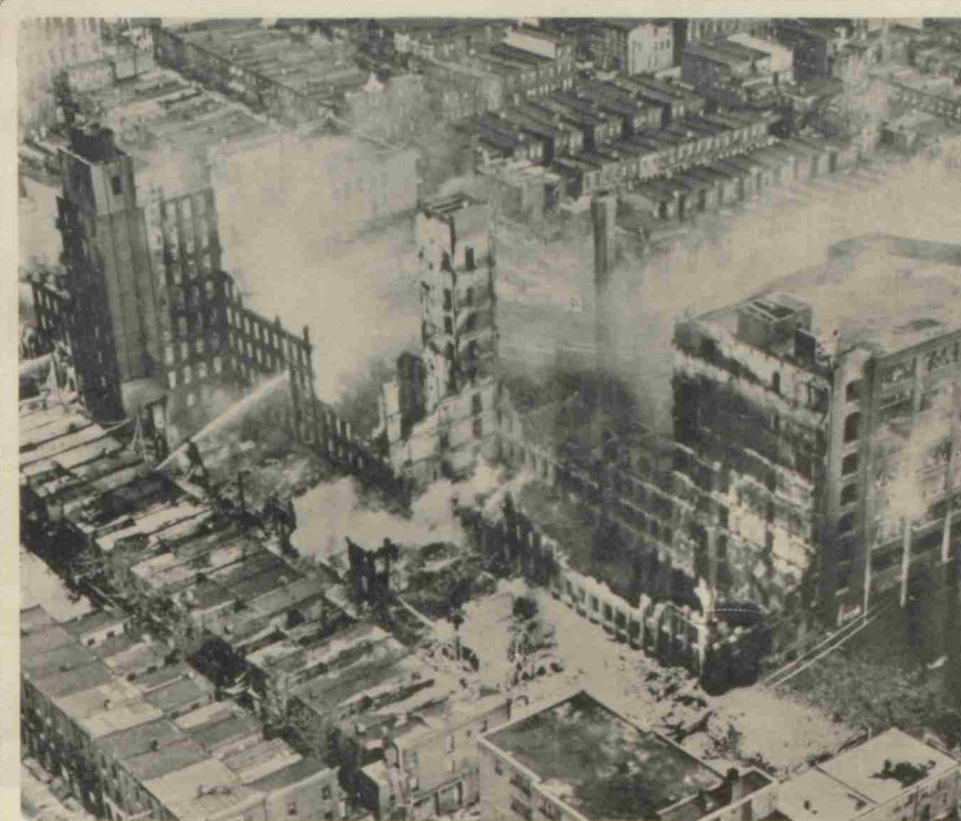
(Above.) PHILADELPHIA, U.S.A. THE SMOULDERING RUINS OF A NINE-STOREY FACTORY BUILDING AND NEIGHBOURING RESIDENTIAL BUILDINGS WHICH WERE CONSUMED BY FIRE ON JANUARY 2. The fire started in the factory and quickly spread to the surrounding houses, where it devastated the homes of some 250 persons. Twelve companies of firemen were called in to fight the blaze which caused extensive damage estimated to run into millions of dollars.
