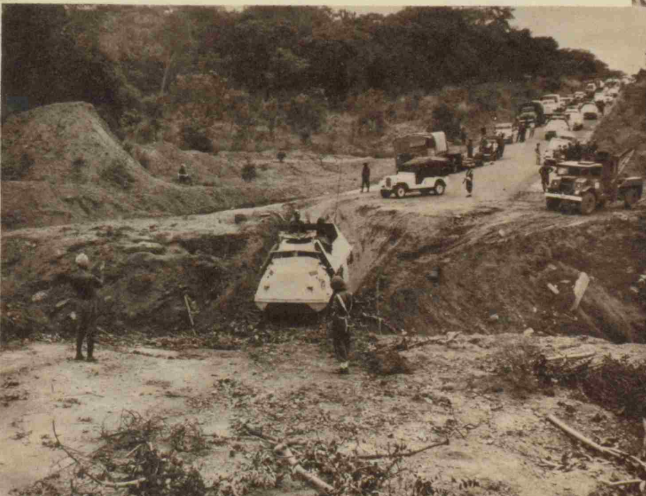
ELEMENTS OF A TWO-MILE U.N. CONVOY NEGOTIATE AN IMPROVISED BRIDGE OVER A CRATER BLOWN IN THE ROAD TO JADOTVILLE. THE KATANGESE SABOTAGED ALL ROUTES TO THE CITY.
