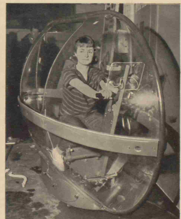
TWO 12-VOLT BATTERIES POWERED THIS "WET" SUBMARINE CALLED THE AQUAMOBILE SUBMARINE.
